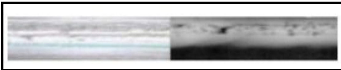
Figure (6-3) Photography of welding sites in metals showing defects that cannot be seen with the naked eye
